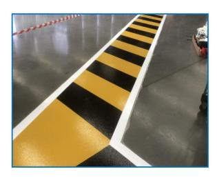
Remove excess flakes or aggregates from the surface by sweeping followed by vacuum. The use of light sanding is recommended for flakes to remove flakes standing proud.
