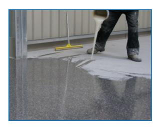
When grouting Pumadur SC, apply using a squeegee pushing well into the surface until saturated then pull back to a tight coat with a short pile roller pre-wetted with Pumadur Grout. Inconsistent application thickness will result in an uneven finish and appearance. The cured product should be protected from other trades using Kraft paper or similar breathable material. Polythene should not be used. Protect the installed floor from damp, condensation and water for at least 4 days.
